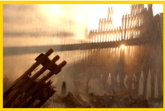
Wreckage from World Trade Center at Ground Zero on September 11, 2001. (Photo Credit: FEMA)
